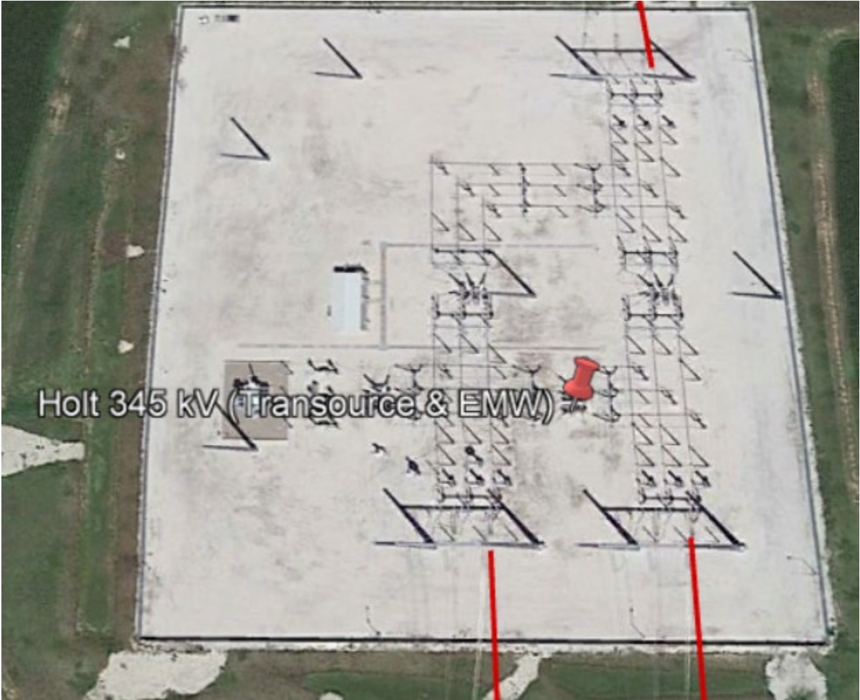
Holt 345kV substation
